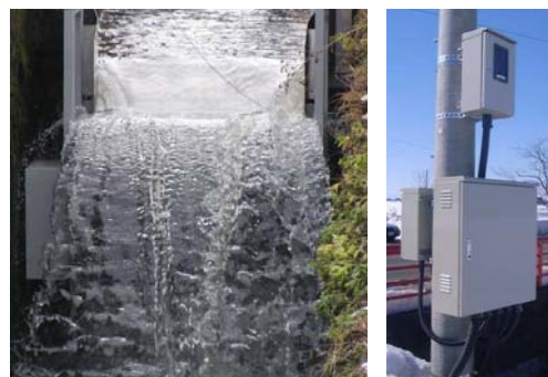
Fig.3 Micro hydraulic turbine installed at drop & power system interconnection equipment
